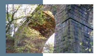
• The former Caledonian Railway Viaduct over the Water of Leith, dates from the late19th Century. It is approximately 250 metres long, 8 metres wide and at its highest point 20 metres above the river. Both arches and buttresses are made up of massive coursed rubble faced stone elements conveying an impression of robust structural strength.
